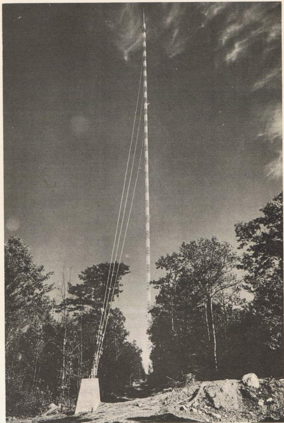
Tallest in the World — TV Tower of WGAN-13, Portland, Maine
