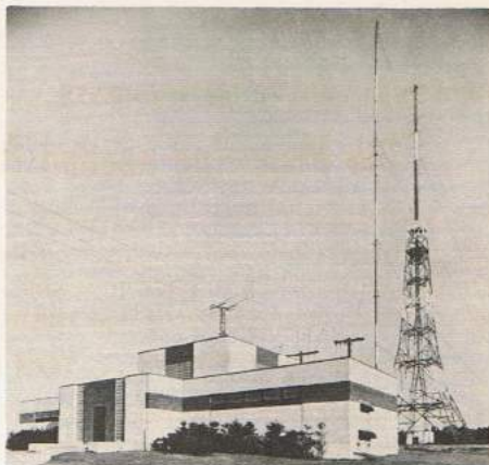
Pioneer FM Station WGTR, Paxton, Mass., in 1941. 10 Bay Turnstyle Antenna at right. This site now used by UHF TV Station WWOR.
