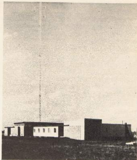
View of the Langata transmitting station of the Kenya Broadcasting Service.
